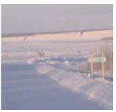
To solve the problem, a thicker ice layer was built on top of the new layer and flooded until the ice thickened enough to support a snow machine, which leveled the rough ice surface.
